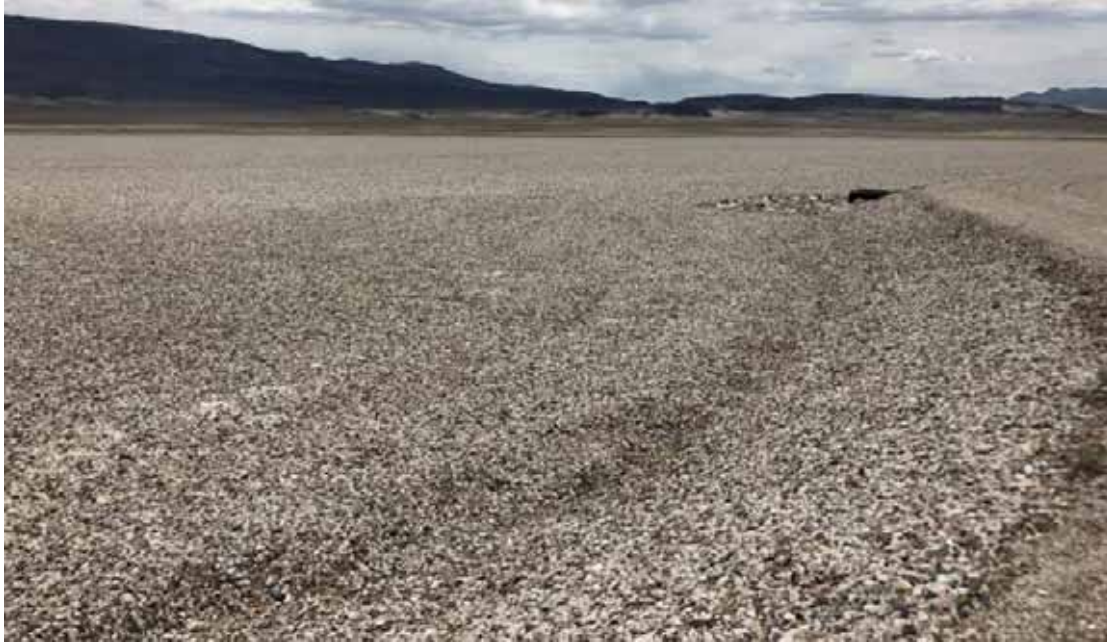
FIGURE 4-9 Dust control using the gravel BACM. SOURCE: Photo courtesy of Stephanie Johnson, National Academies.
