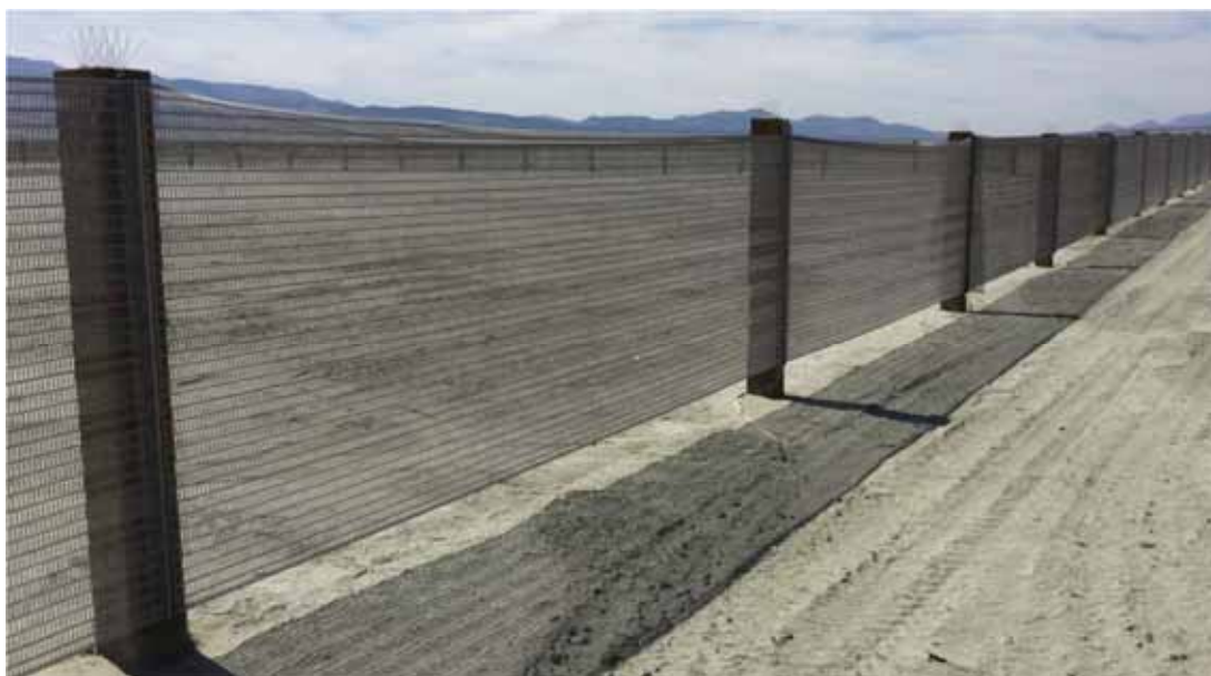
FIGURE 4-13 Sand fence at Owens Lake. SOURCE: Schaaf, 2019.
