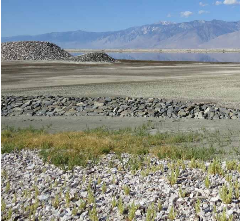
FIGURE 4-12 Use of cobbles and boulders at Owens Lake as part of the Land Art Project, with cobbles used along trails to provide enhanced public access. The cobbles trap seeds and sand, providing sites for the establishment of native vegetation.
