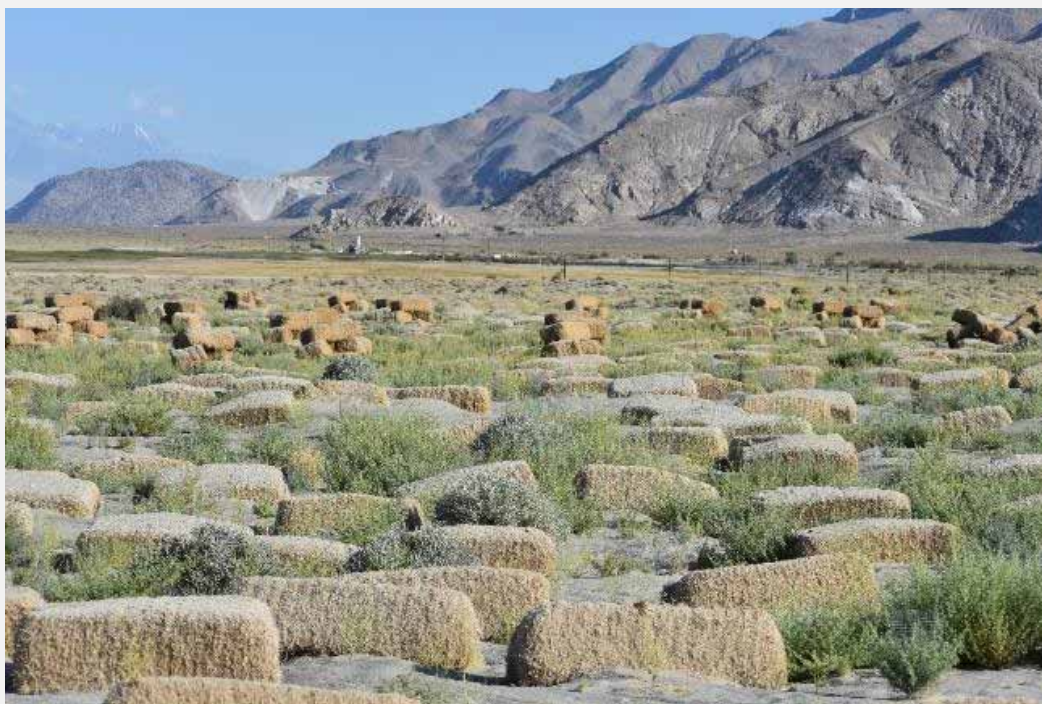
FIGURE A Use of solid natural roughness elements at the Keeler Dunes. SOURCE: Photo courtesy of David Allen, panel member.
