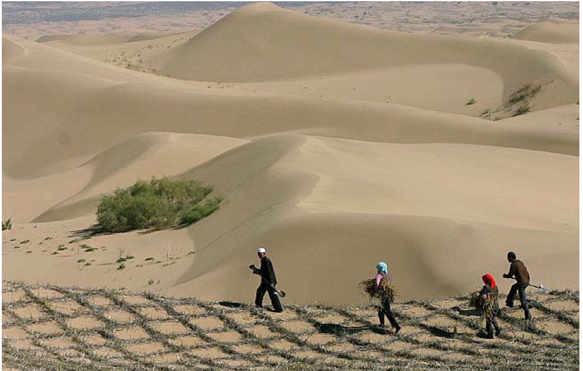
Installing straw checkerboard in stabilized belt of dune, Tengger Desert, China
