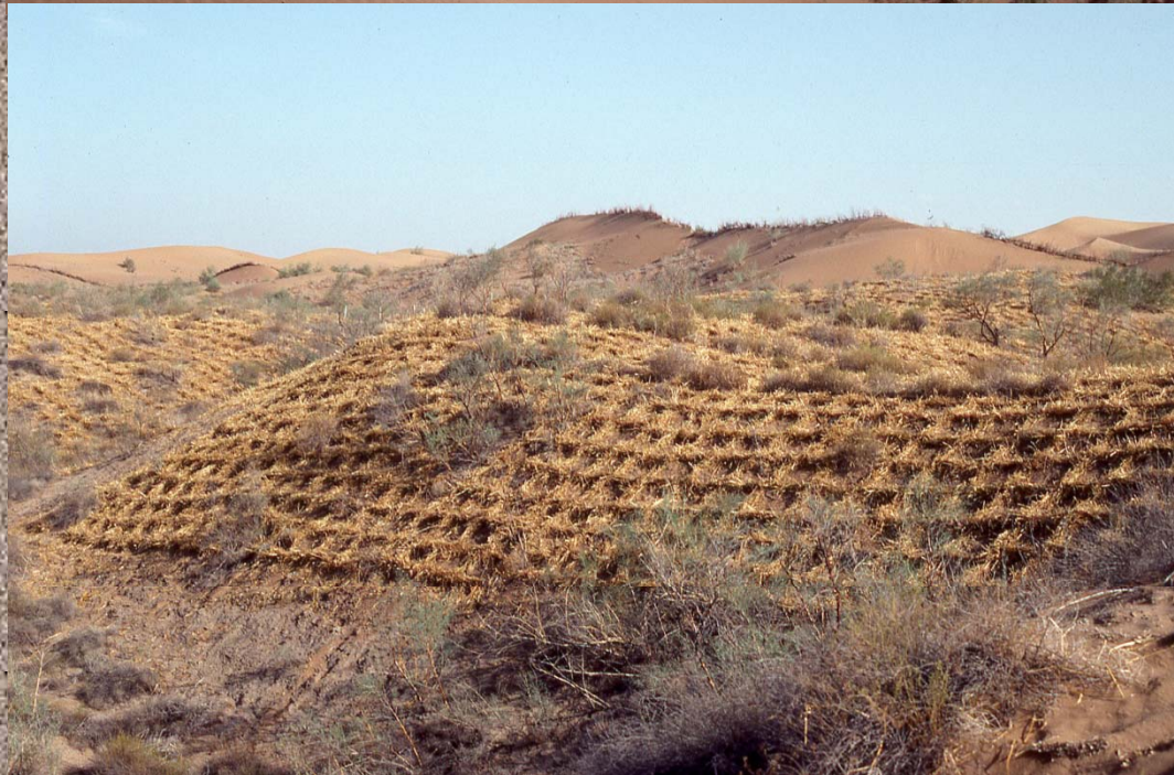
Straw Checkerboards Shapotou, China
