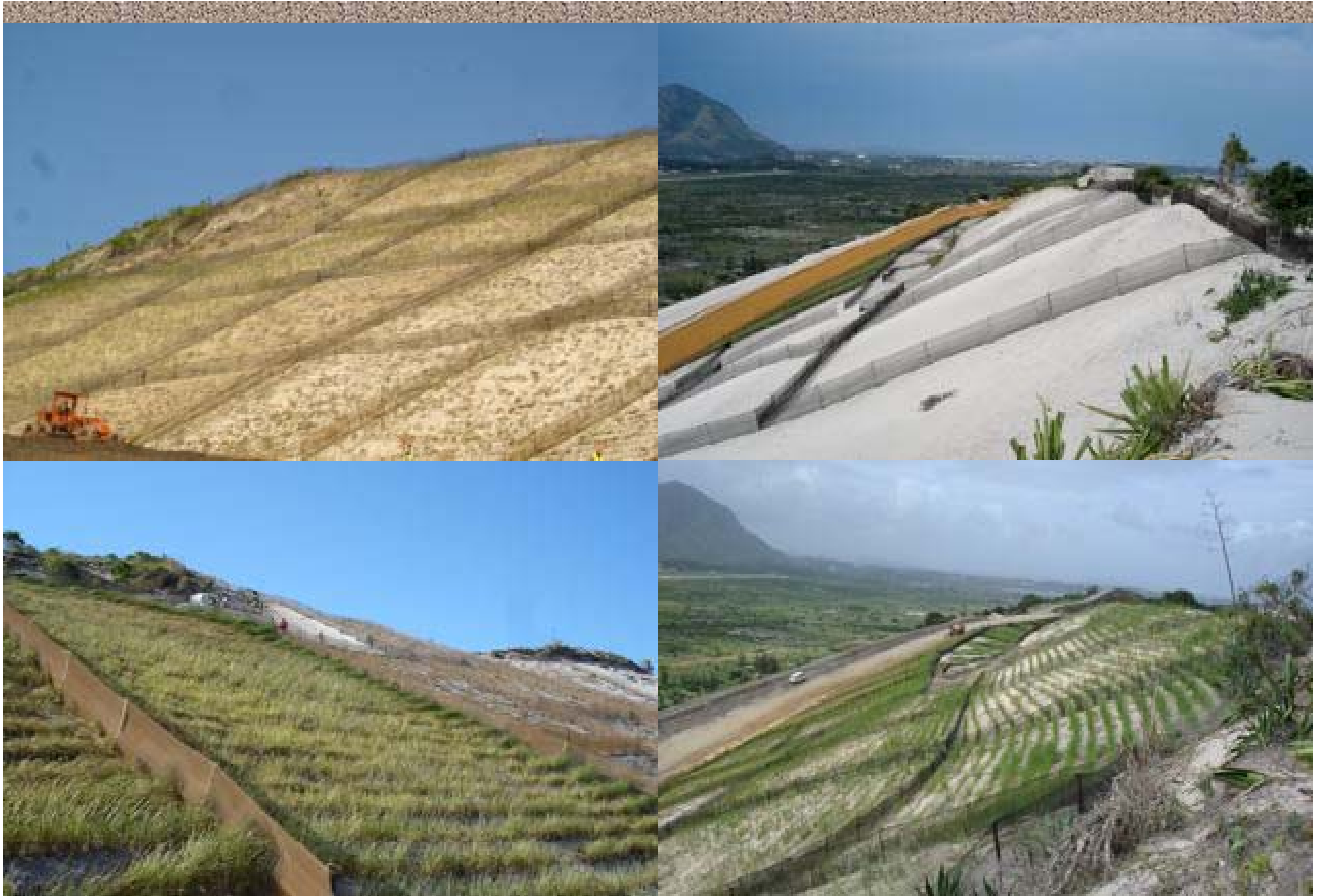
Dune stabilization with fences and grass, Madagascar.
