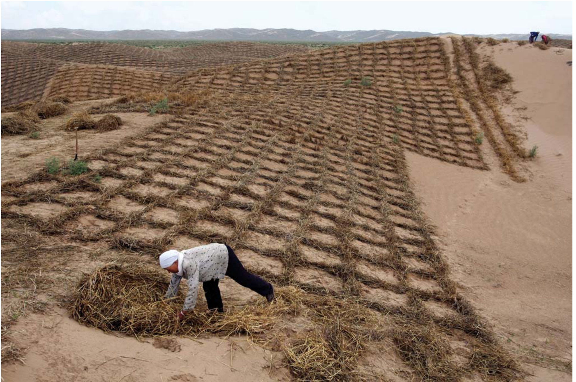
Installing straw checkerboard, Tenggar Desert, China
