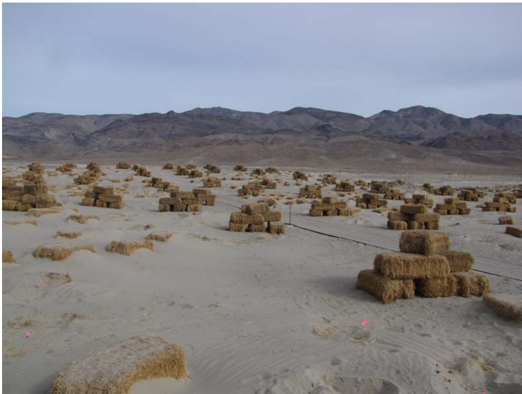
Figure 6. Newly constructed bale mounds in the Southern Dunes. View to the east.
