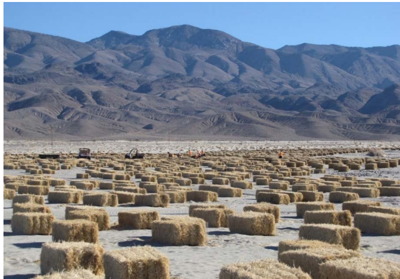
Figure 6-5: Straw Bale Array in the Keeler Dunes Dust Control Project (January 2015)
