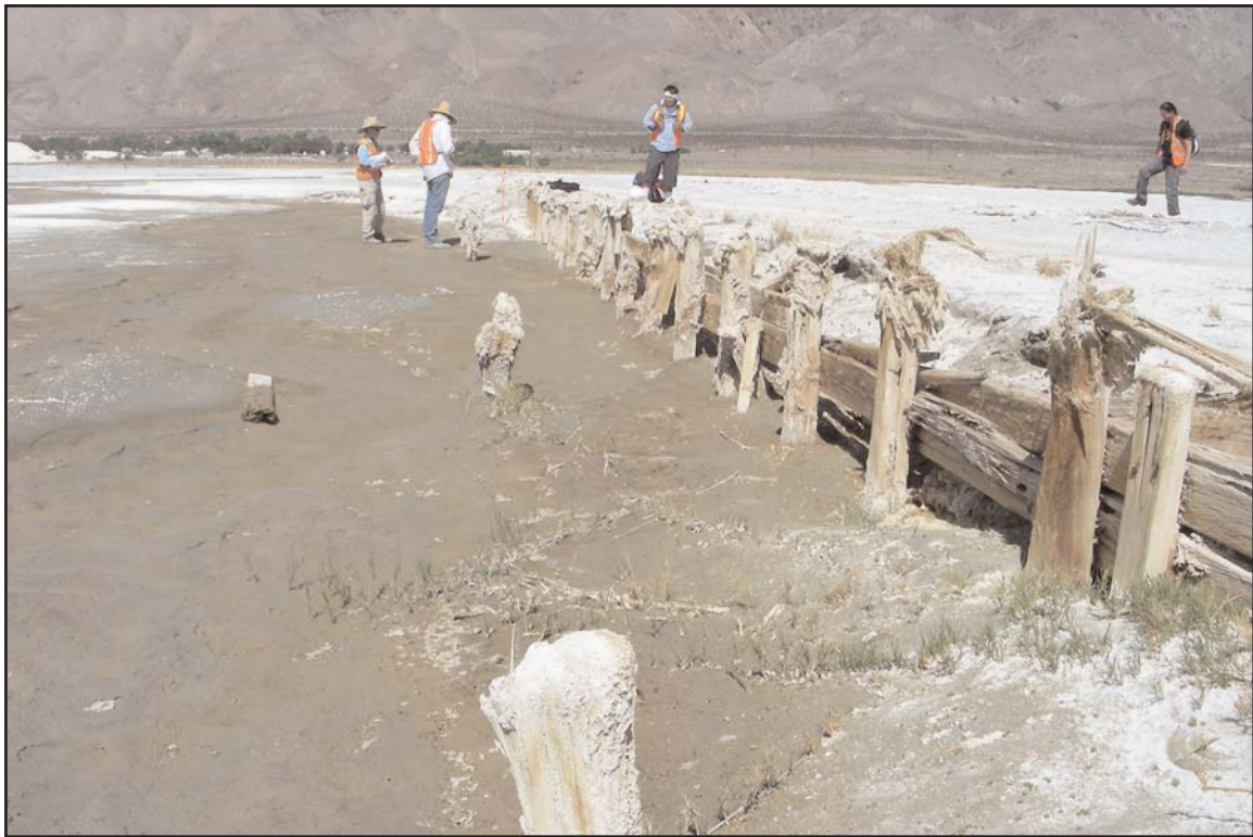
PHOTO 1 Overview of Section 1, looking west
