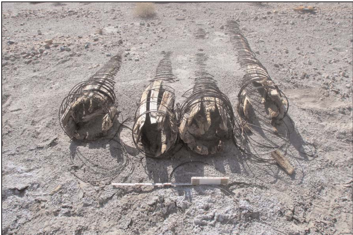
PHOTO 2 Wooden culvert
