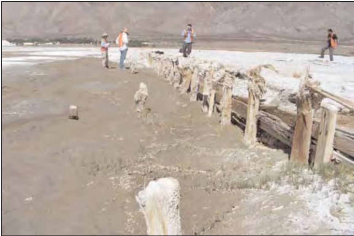
PHOTO 1 Overview of Section 1, looking west
