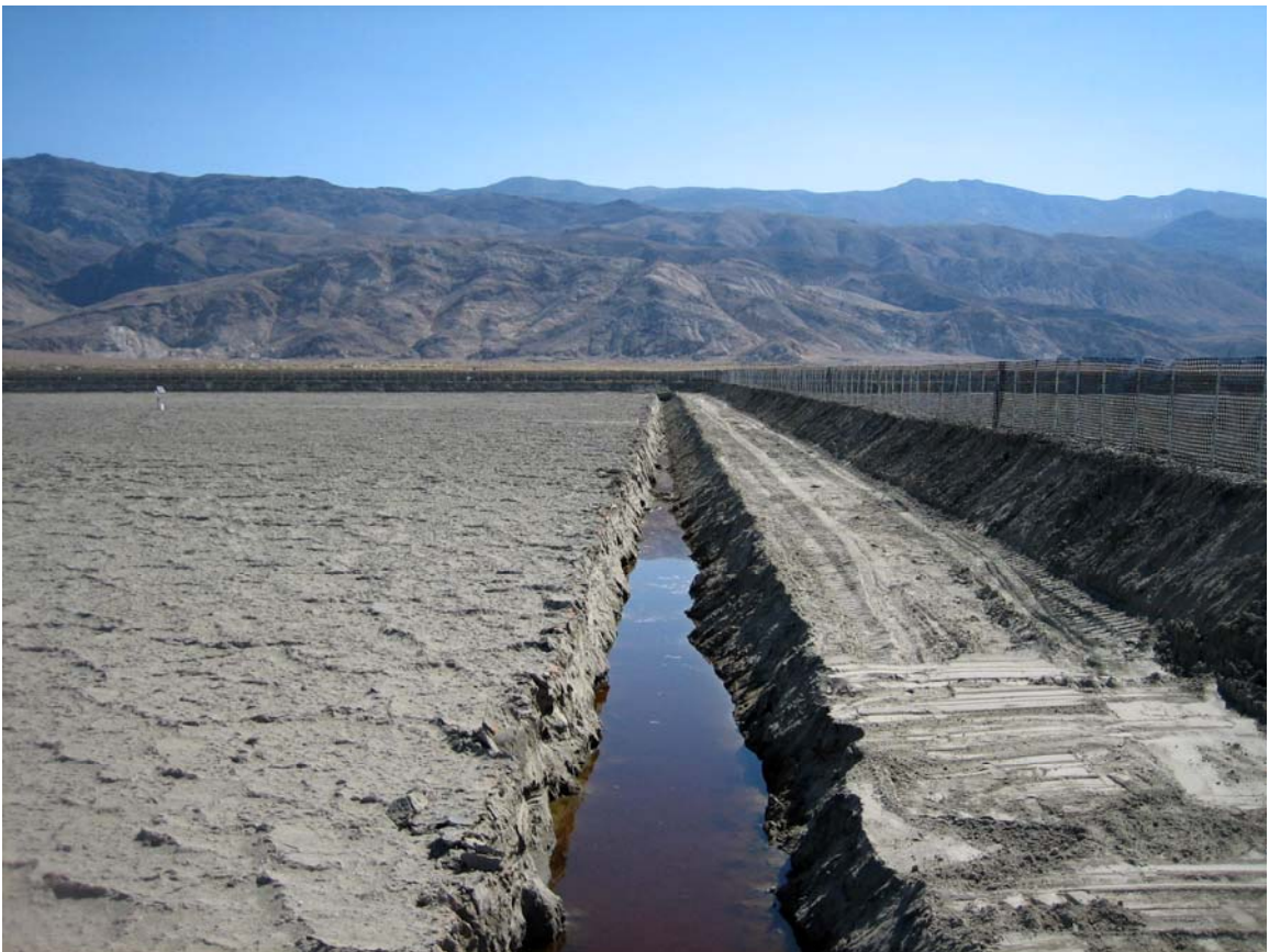
Figure 5.18 – Moat and Row test – ground level view
